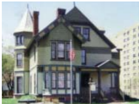
THE HERRICK HOUSE ON UNION AVENUE WAS SAVED FROM DEMOLITION AND ADAPTIVELY REUSED AS THE PEEKSKILL MUSEUM IN 1976.
